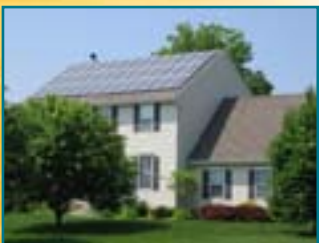
Solar panels on the roof
